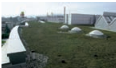
Commercial Building Enterprise, Sursee, Suecia
